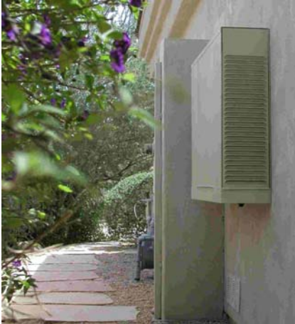
Figure 2. Adobe's new through-the-wall evaporative cooler
