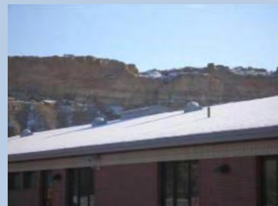
Solatubes (shown on roof) provide daylight to interior spaces at Greybull Elementary Photo: SWEEP
