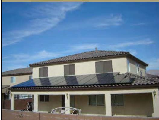
5 KW residential roof mounted system
