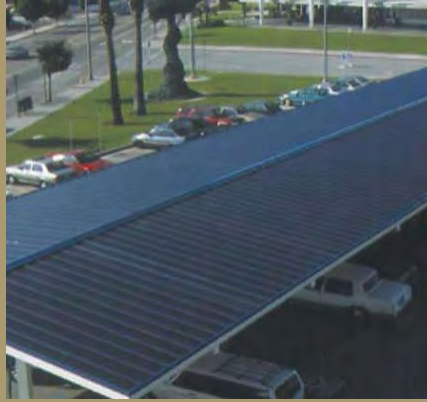
Thin Film installed on Parking Structure
