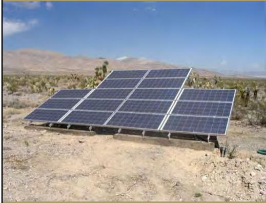
3 KW Fixed ground mounted system in remote location
