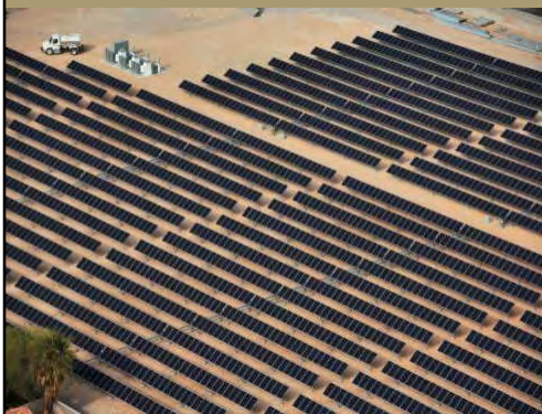
800 KW Tracking ground mounted system at Ronzone Reservoir
