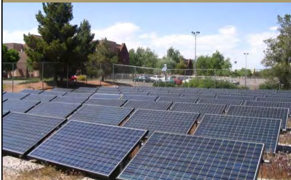
20 KW Fixed ground mounted system at UNLV (15 years old)
