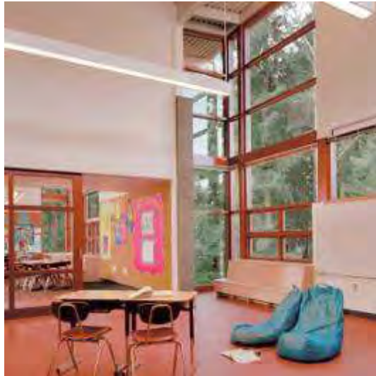
Ceiling fans and operable windows to maximize daylight and natural ventilation
