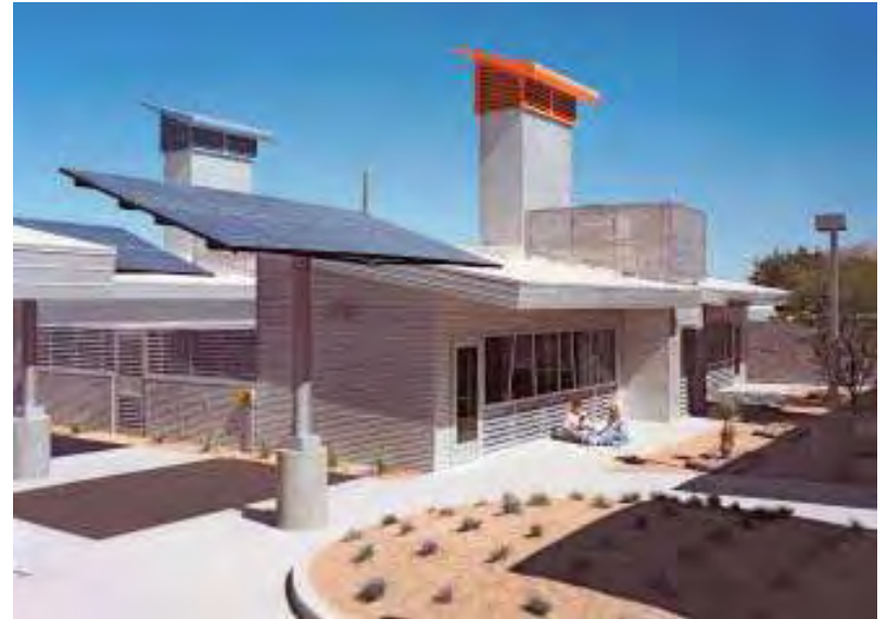
Back-up power supplied by PV
