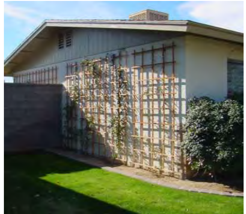
Exterior Shading devices
