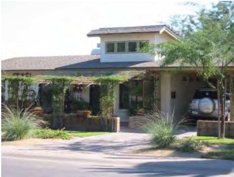
Shaded Entry Courtyard
